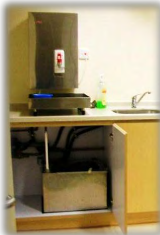
Used boilers, sinks and sump pump systems were reused in pantries of NSB
