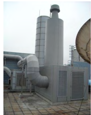
Newly installed fume extraction fan LCF-35 on the roof of Blue Zone, AC1
