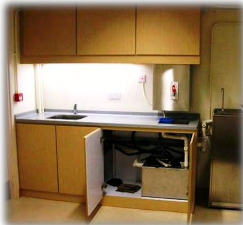
Used boilers, sinks and sump pump systems were reused in pantries of NSB
