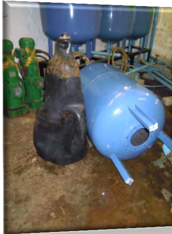
300L pressure vessel of Floor 7, AC1 kitchen fresh water tank diaphragm repaired
