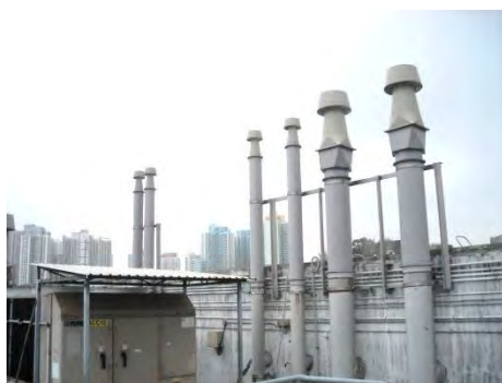
Newly installed jet nozzles on the roof of Purple Zone, AC1
