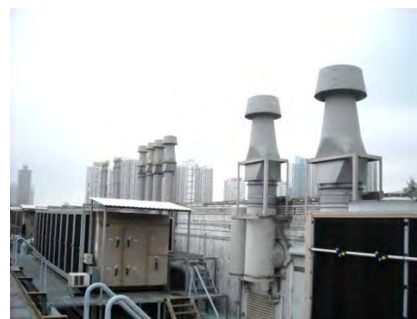
Newly installed jet nozzles on the roof of Purple Zone, AC1
