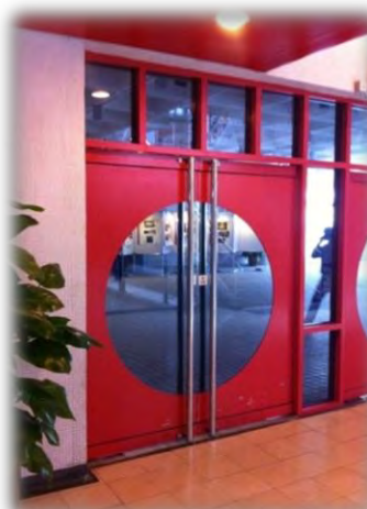
Used glass doors were reused at entrance to U-Concourse on Floor 4, AC1 to replace the damaged ones
