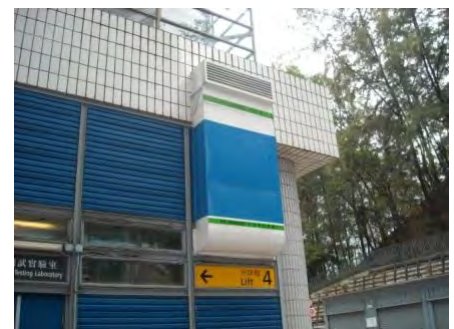
Extended fresh air intake louver to upper location outside 1SC04
