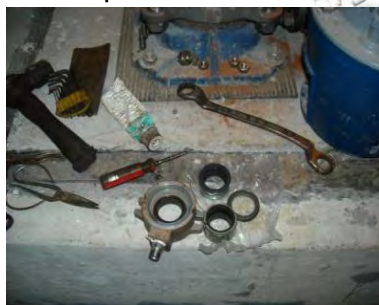
Ball valve serving AC2 kitchen fresh water tank reconditioned
