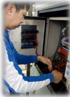
The defective electronic control cards of chillers at AEB rooftop, AM Building, CMC & AC2 were retrofitted.
