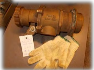
Ball filling valve of roof fresh water tank of AM Building was overhauled
