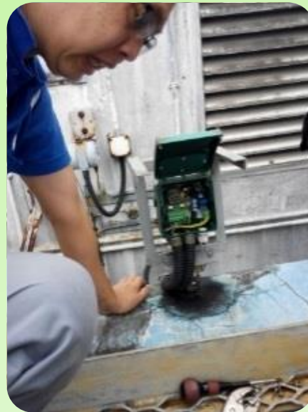
A printed circuit board from a defective flow rate sensor of a chiller in Green Zone, AC1.
