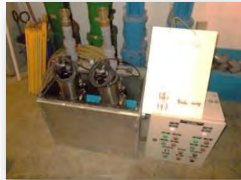
Sump pit submersible pumps / control panels / fittings from AC3
