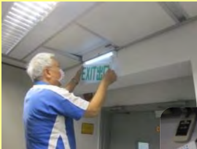
Failed LED light stripes of 285 nos. of EXIT light boxes at AC1, CYC Building, FYW Building, MMW Building public corridors were replaced, instead of replacing the whole EXT light boxes
