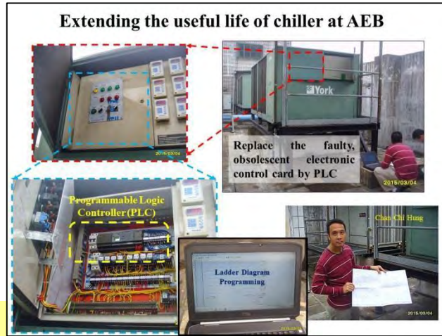
The defective electronic control cards of chillers at AEB rooftop, AM Building, CMC & AC2 were retrofitted.
