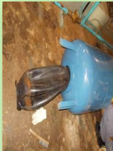
300-litre pneumatic pressure vessels from pump room of Student Residence
